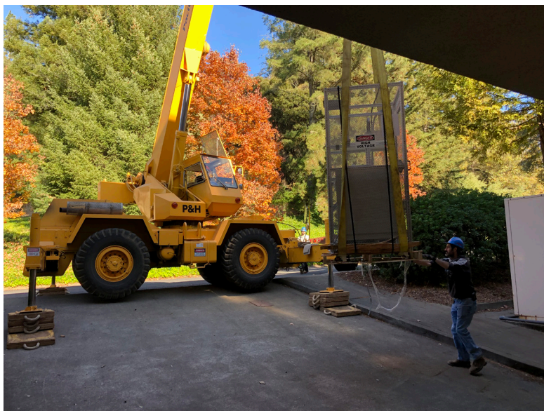
Members of the facilities crew move the high voltage cage for the ORNL equipment into position for unloading.
